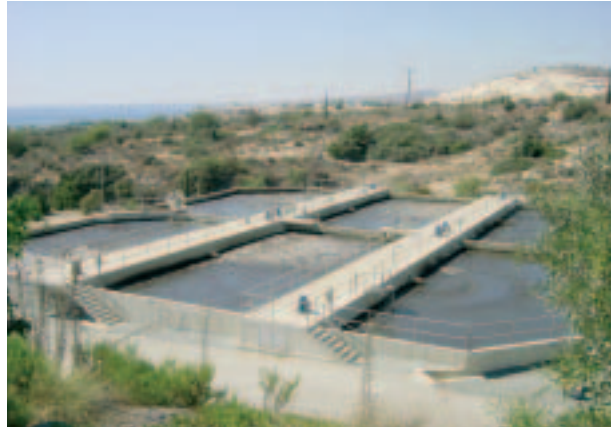
CYPRUS | Wastewater treatment plant near Limassol
