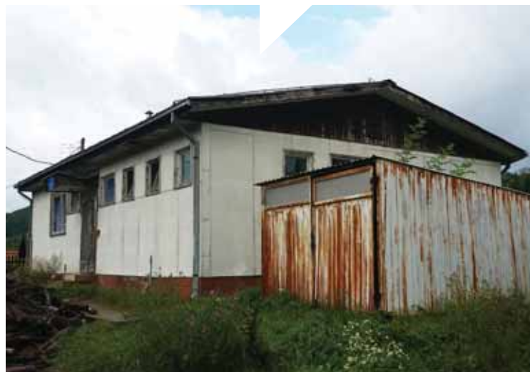
Left: A care centre before restoration
