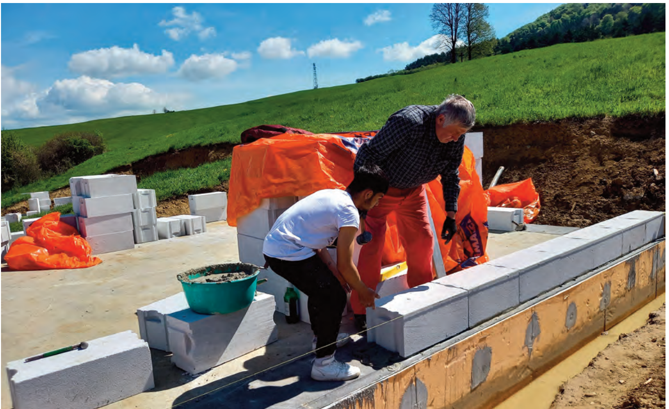
Construction of homes as part of the HERO project.
