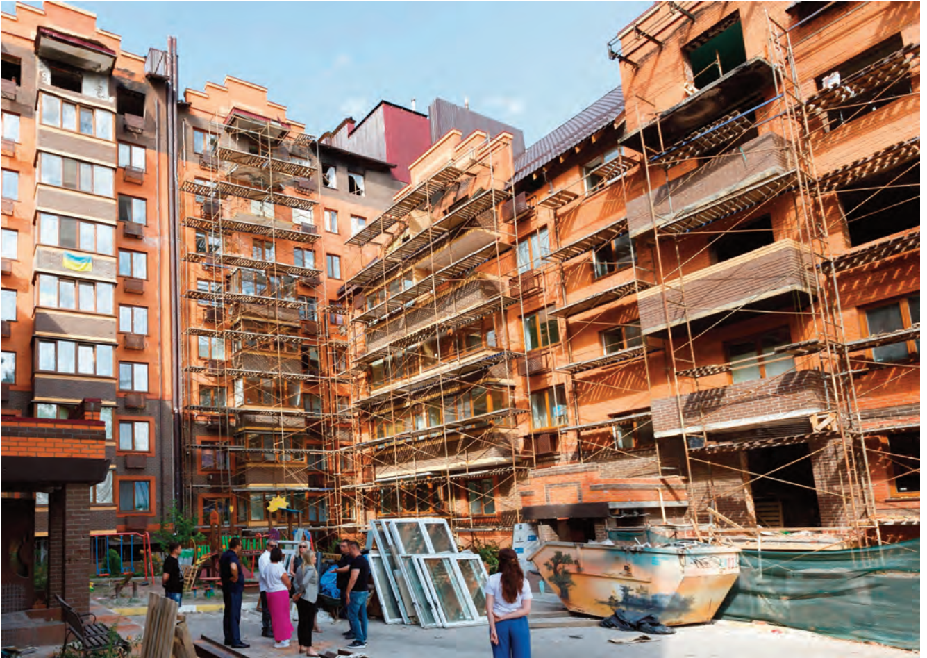
Rehabilitation works of war-damaged buildings underway in Ukraine.
